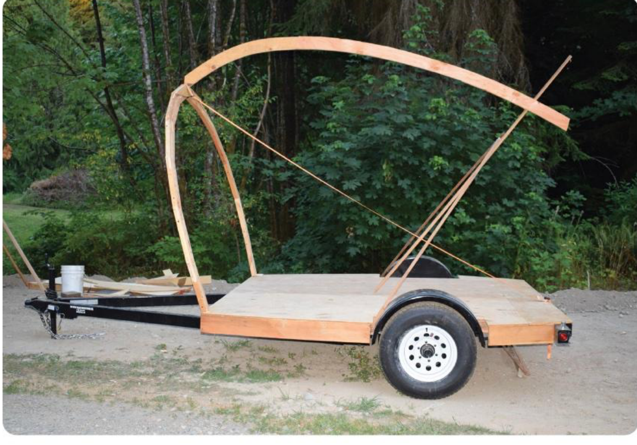
The first template for the ridge member. I used this template to build a stout ridge beam out of Douglas Fir. From this side perspective you can better see the angle of the front wall.
